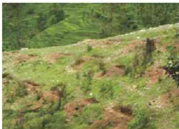
Contour Trenching at Badgaon, Alaknanda Soil Conservation Forest Division, Gopeshwar in 5 ha area in FY 2016-17.
